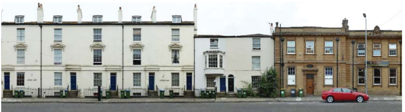
10-1 Latimer Gate, Bernard Street Grade II Listed
