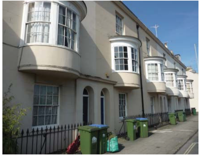
Wheelie bins on the street undermine the quality of the buildings and overall townscape
