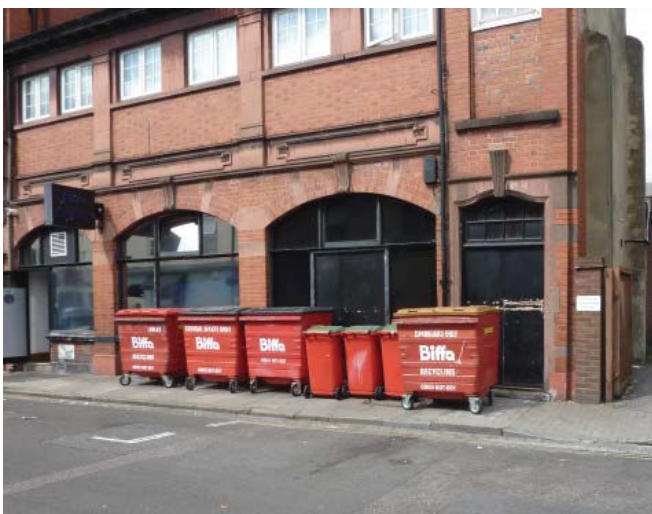
Commercial waste bins on the footway are a visual nuisance and obstruction, John Street
