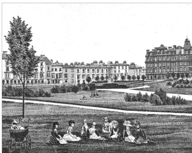
Figure 17: Late Nineteenth century Queen's Park
