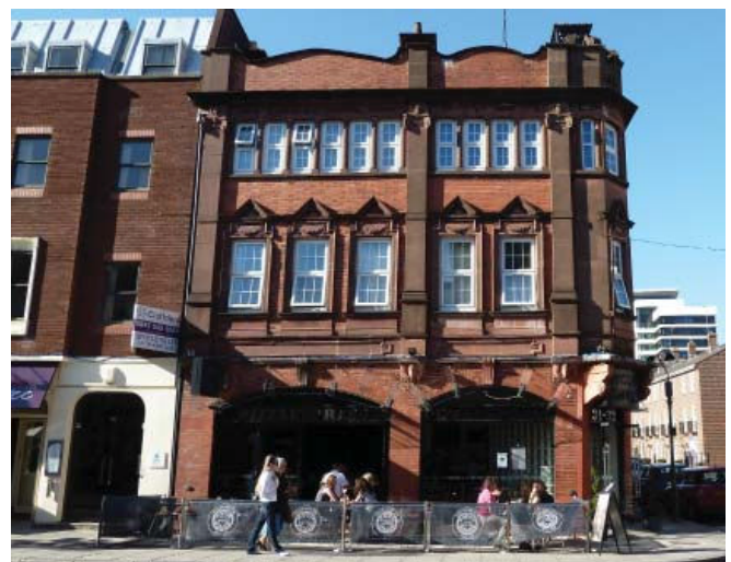
Good detailing undermined by the use of uPVC windows, 31 and 32 Oxford Street
