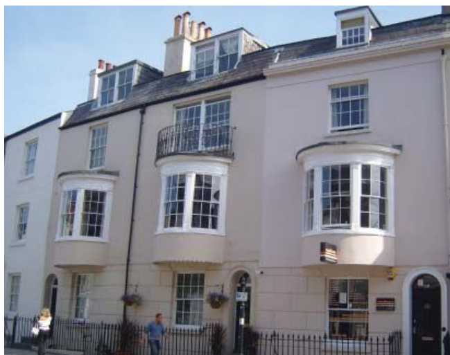
Fine distinctive semi-circular bow windows, Oxford Street
