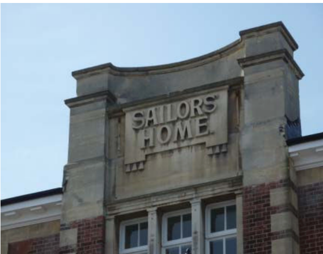
Stone motif on the surviving facade of the former Sailor's Home, Oxford Street
