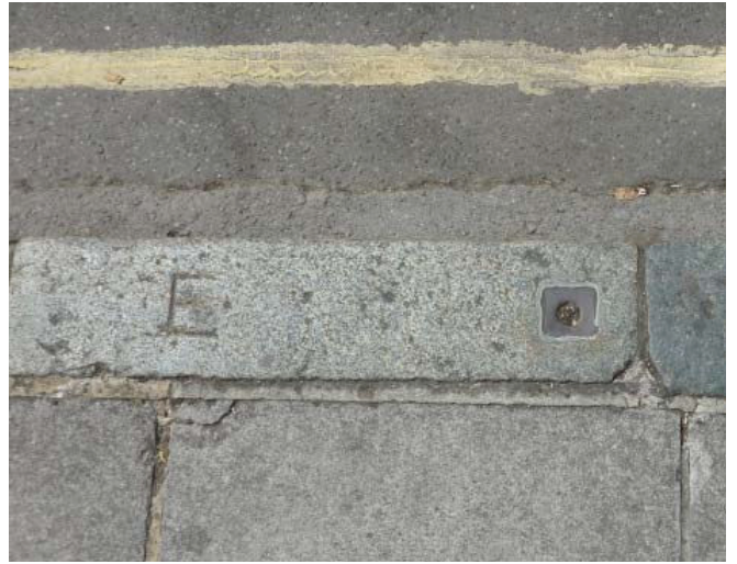
Granite kerb stone and steel socket used to hold up a shop front canopy, Oxford Street
