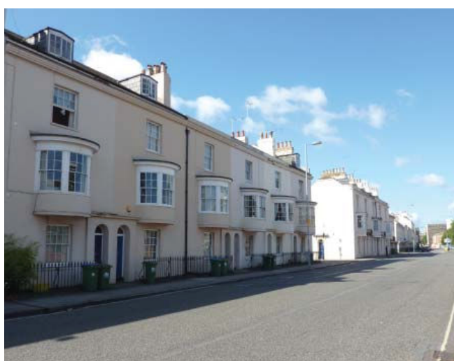
Nineteenth century terraced town houses, Bernard Street
