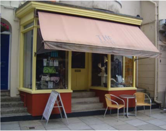
Intact historic shop front, 24 Oxford Street
