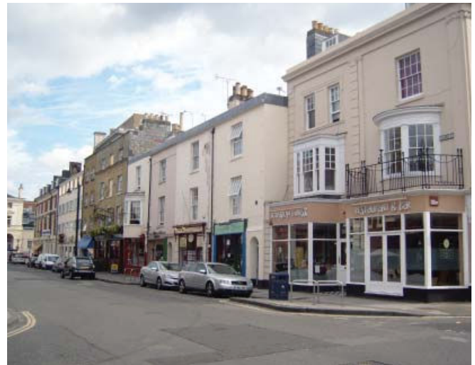
Mixed uses along Oxford Street
