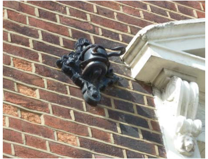
Cast iron tram rosette on the wall of The Court Jester public house, Terminus Terrace
